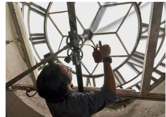
Each day, Mohd Rashidi and his fellow team members will spend three hours here to wind the clock, clean as well as oil the mechanism.
